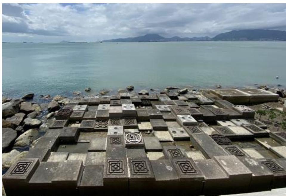
Example: Eco-shoreline at Tung Chung (bio-blocks)
