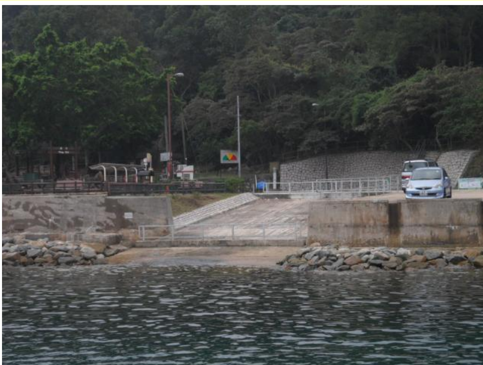
Example: Wong Shek Slipway
