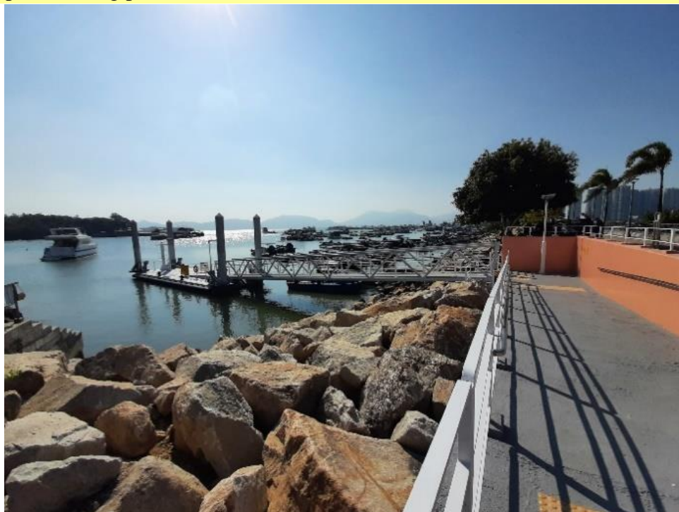
Example: Floating pontoon at Tuen Mun Area 27
